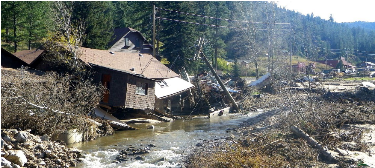
Figure 72: Impacts of the Front Range Flood on West Creek in Glen Haven, Colorado (September, 2013). At this location, the flood was not extreme ( E_f = 1.40 ; Q = 7300 cfs < Q_{mf} = 8200 cfs), but the impacts on the community were catastrophic.
